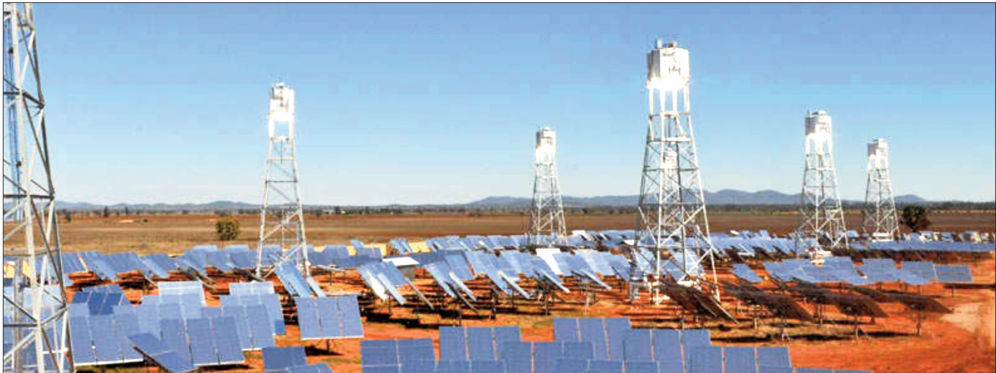
Graphite Energy's Lake Cargelligo facility.
